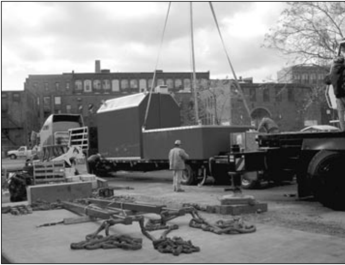
A crane prepares to lift the emergency backup generator into position.
