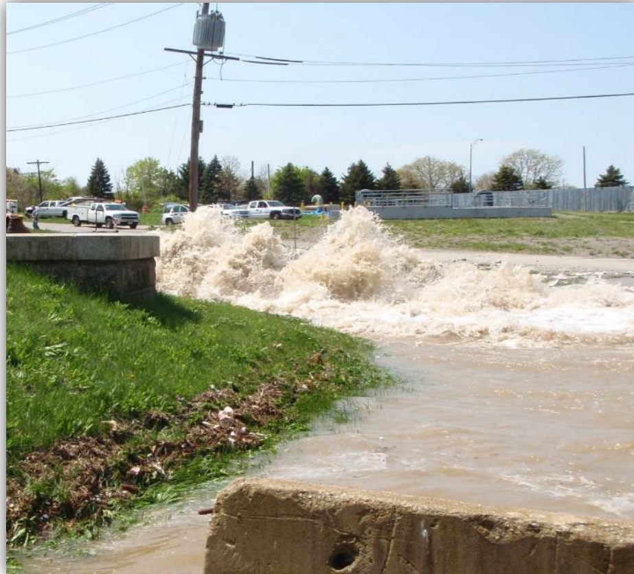
250 MGD flow at Shaft 5 break....
