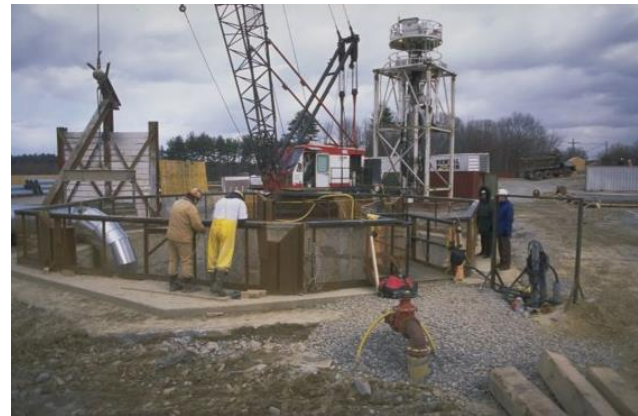
Example of shaft construction activity
