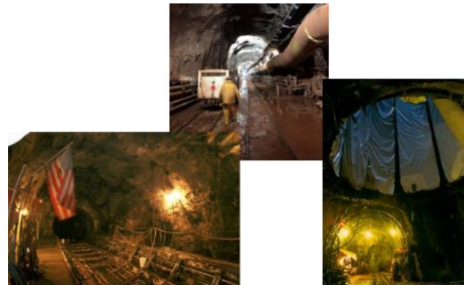
Example of tunnel boring activities
