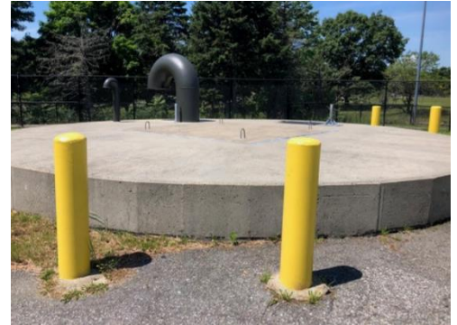
Example of final conditions of a shaft
