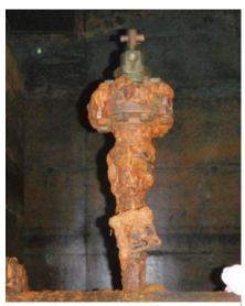
Corroded air valve at Shaft 9A
