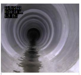
WASM 3 Cleaned and Lined Piping
