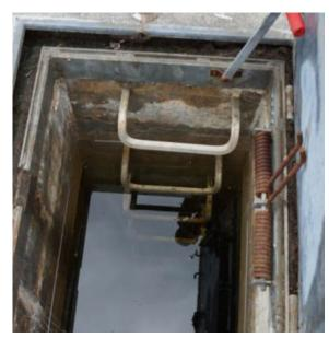
Flooded Shaft 7D valve chamber
