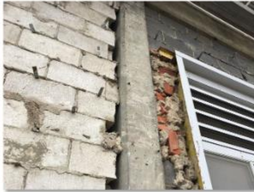
Figure 2 - Headworks Siding Removed
