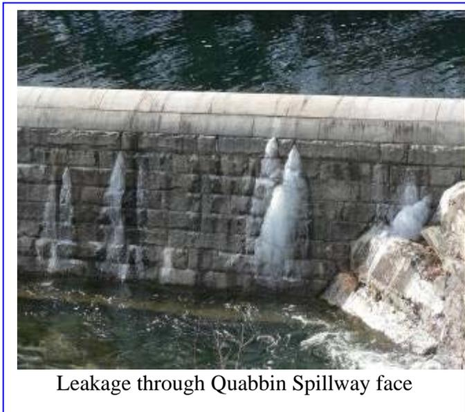
Leakage through Quabbin Spillway face
