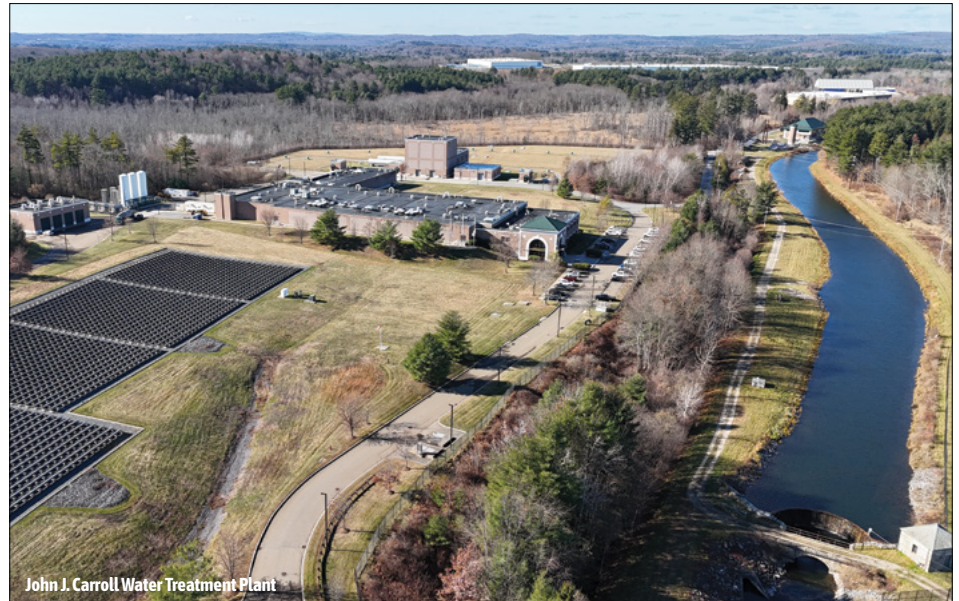
John J. Carroll Water Treatment Plant
