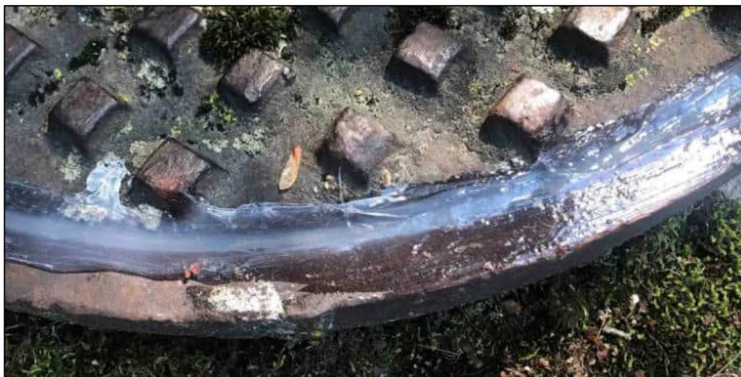
Figure 3-1. Example of a Silicon Seal on the Manhole Cover to Prevent Odors from Escaping
