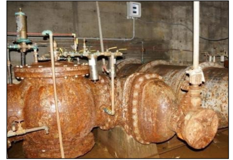
Tunnel Valves in Need of Repair
