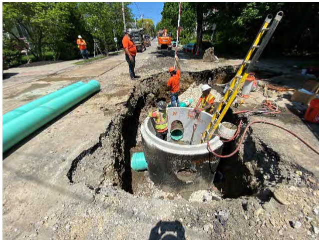
Additional Drain Relocation on Russell Avenue
