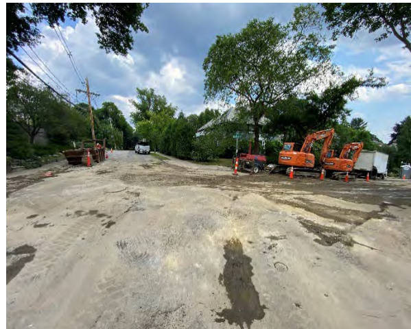
Numerous Trenches on Bellevue Road
