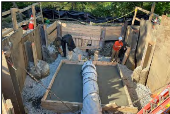
Charles River Leak Repair
