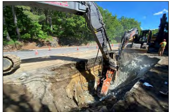
Ledge Removal in Waltham
