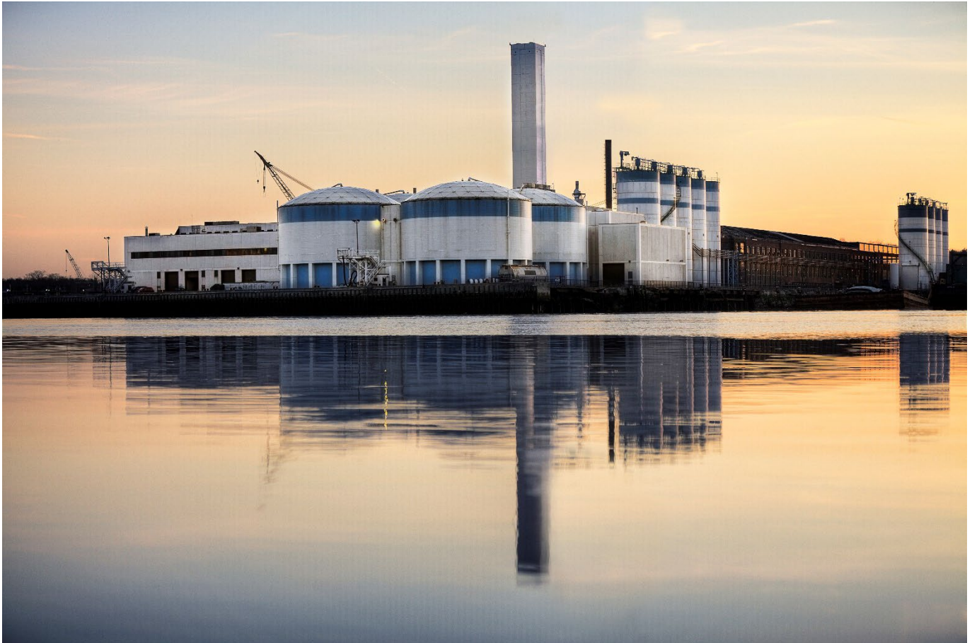
MWRA Sludge Pelletizing Facility
