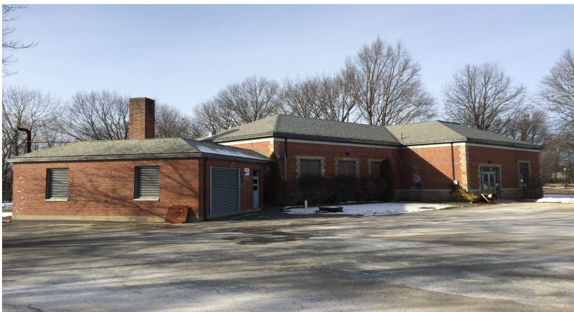
Alewife Brook Wastewater Pump Station
