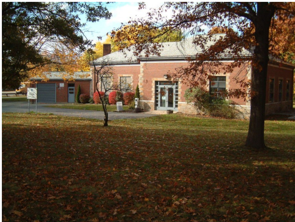
Alewife Brook Wastewater Pump Station
