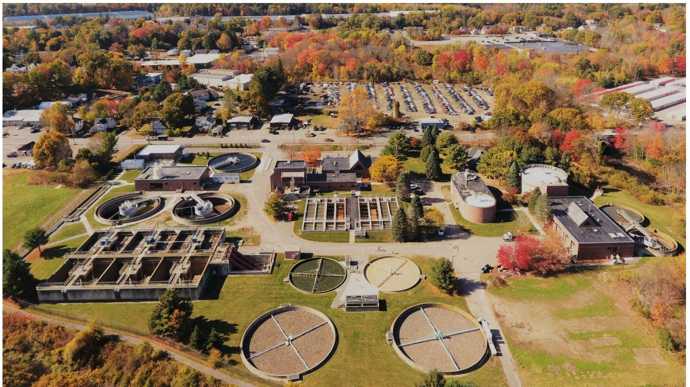
Clinton Wastewater Treatment Plant
