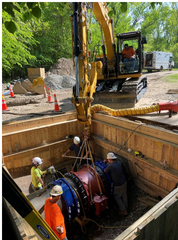
Shaft 7C Main Line Valve Replacement
