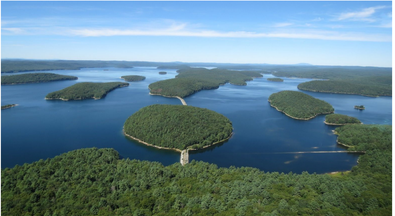
Baffle Dams Quabbin Reservoir
