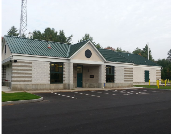
Brutsch Water Treatment Facility
