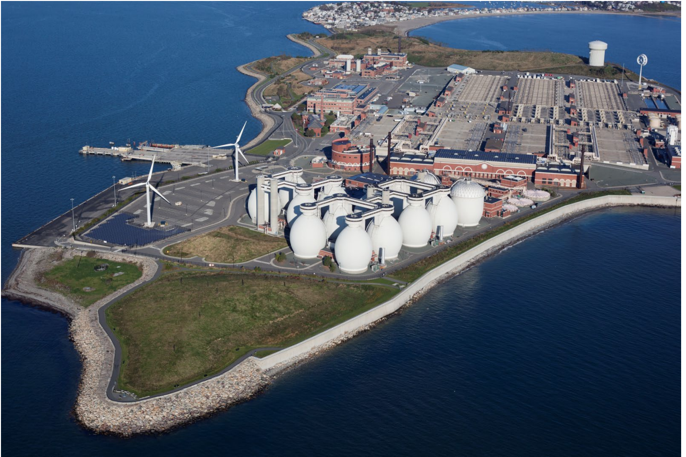
Deer Island Wastewater Treatment Plan
