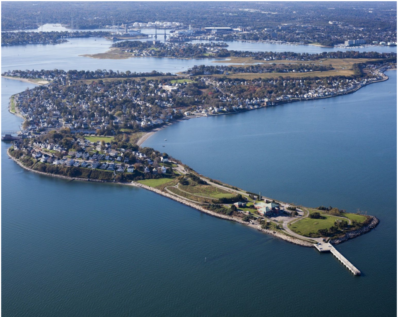
Nut Island Headworks
