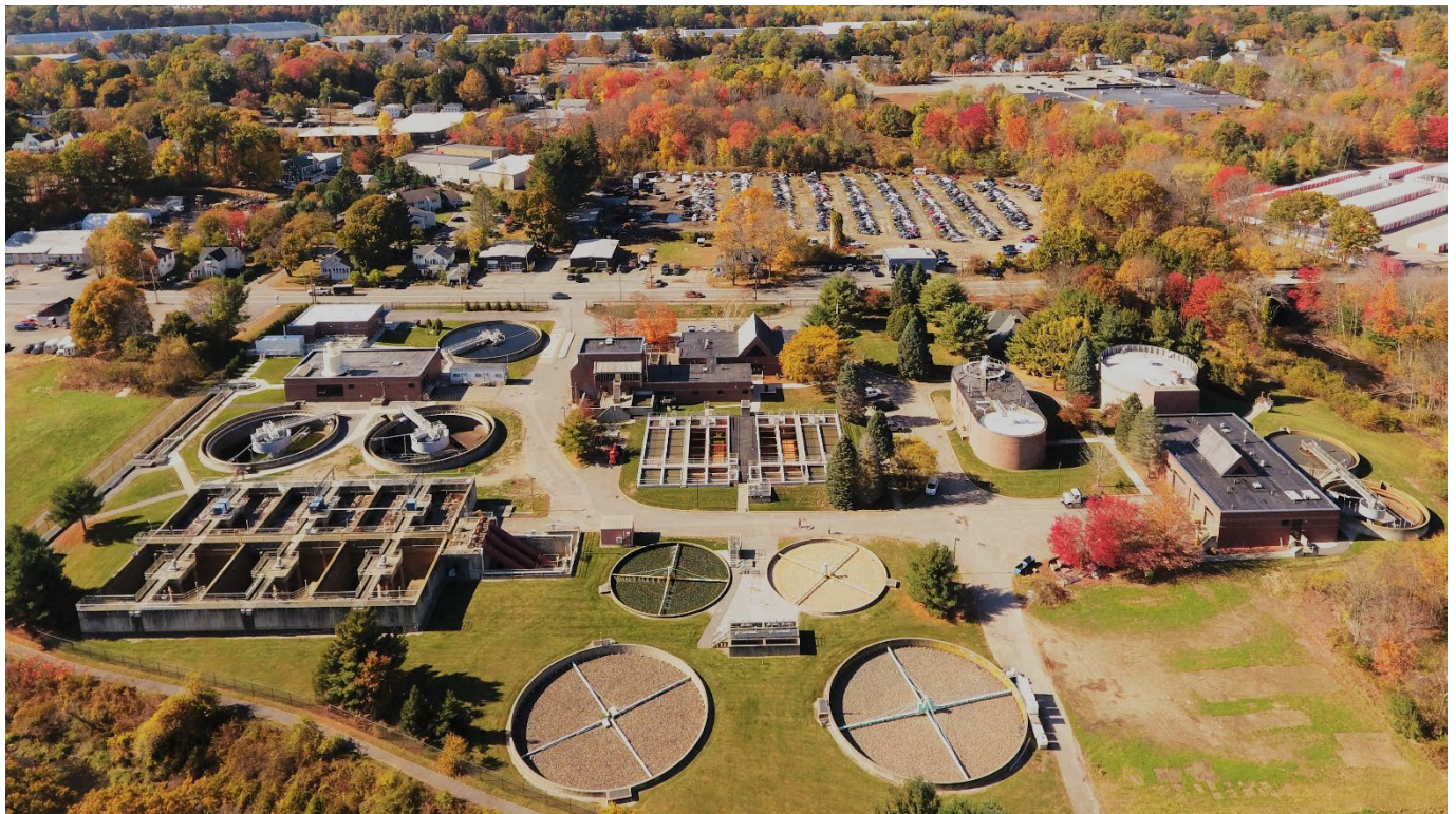
Clinton Wastewater Treatment Plant
