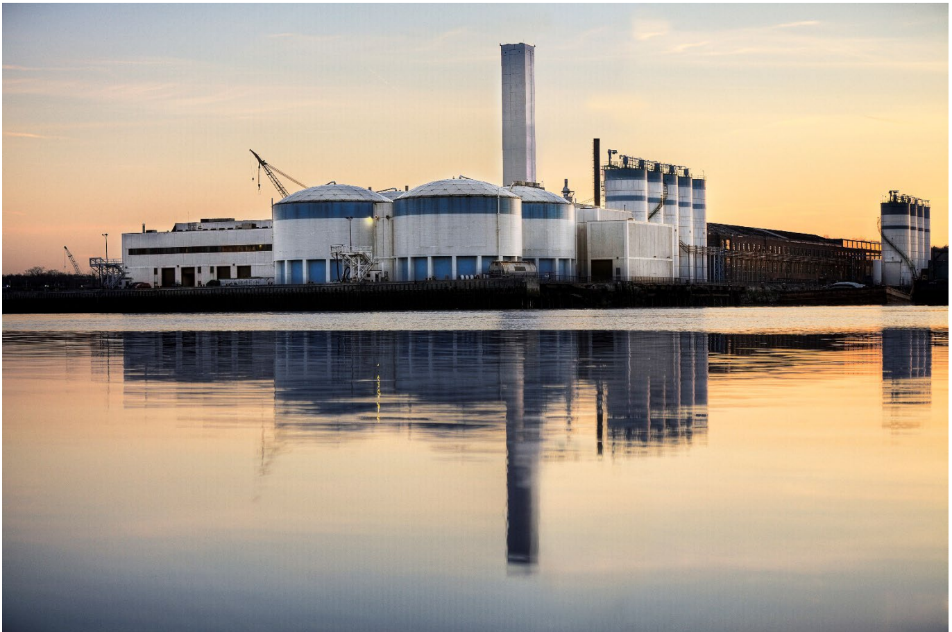
MWRA Sludge Pelletizing Facility
