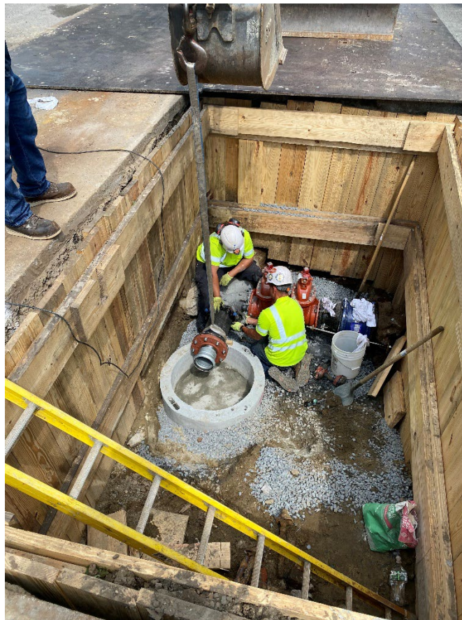
Blow off valve replacement in Dedham
