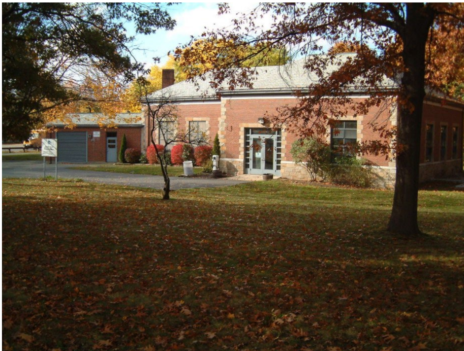
Alewife Brook Wastewater Pump Station
