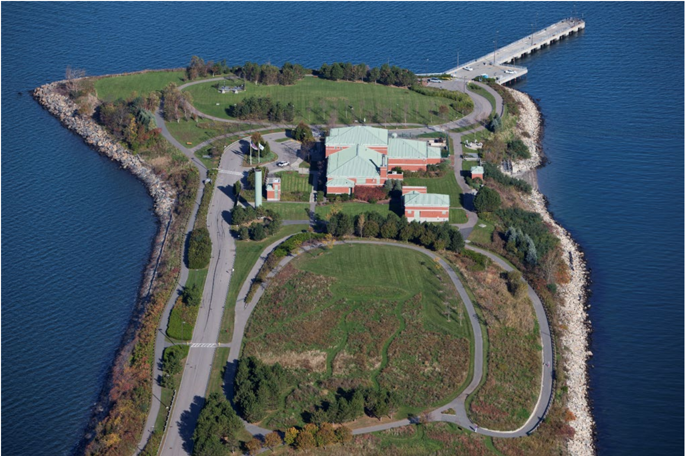
Nut Island Headworks
