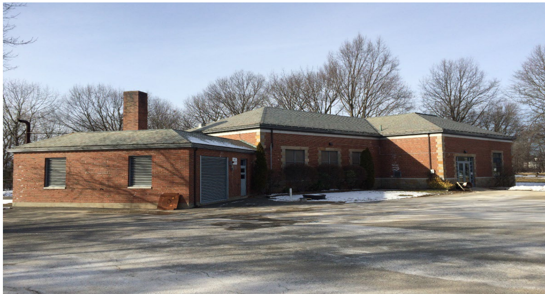
Alewife Brook Wastewater Pump Station
