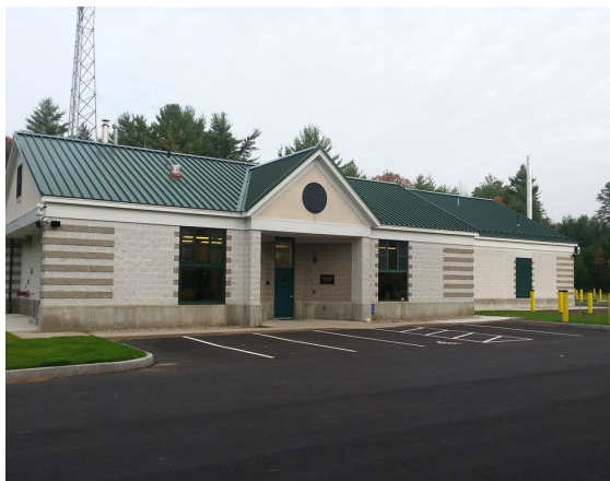
Brutsch Water Treatment Facility
