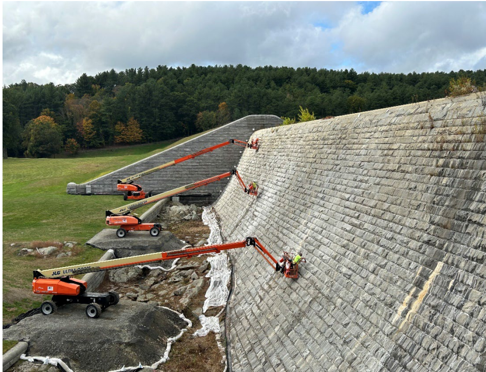
Sudbury Dam Repointing
