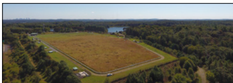
Norumbega Covered Storage Facility in Weston
