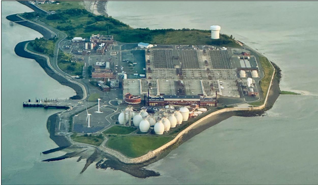
Deer Island Wastewater Treatment Plant
