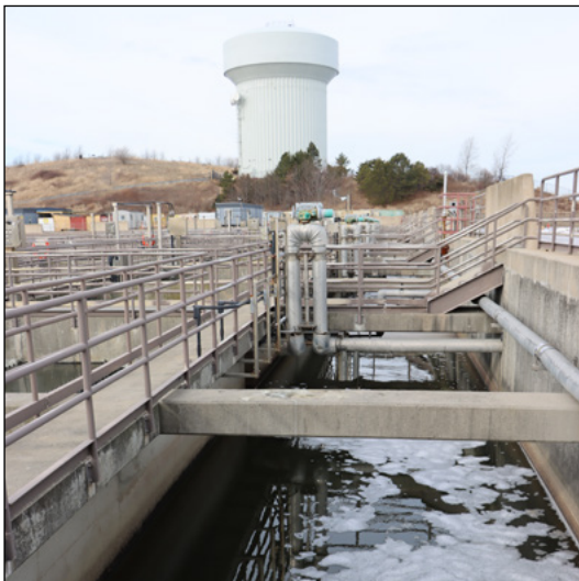
Deer Island Wastewater Treatment Plant
