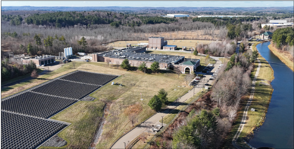
John J. Carroll Water Treatment Plant
