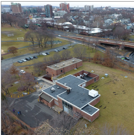
Cottage Farm CSO Facility
