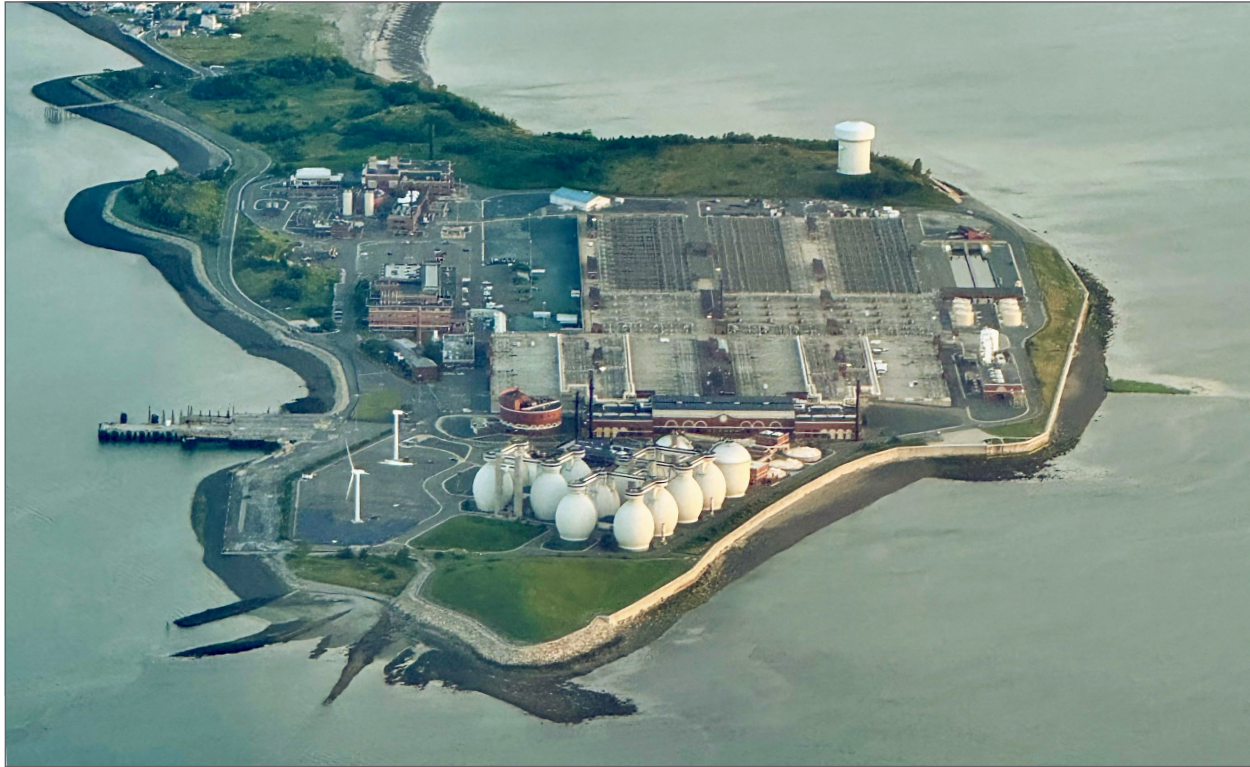
Deer Island Wastewater Treatment Plant
