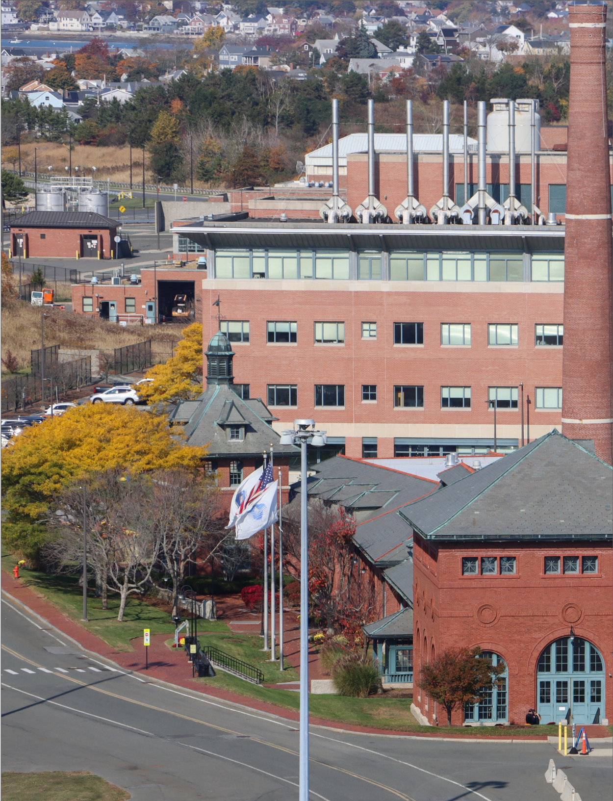
Deer Island Wastewater Treatment Plant
