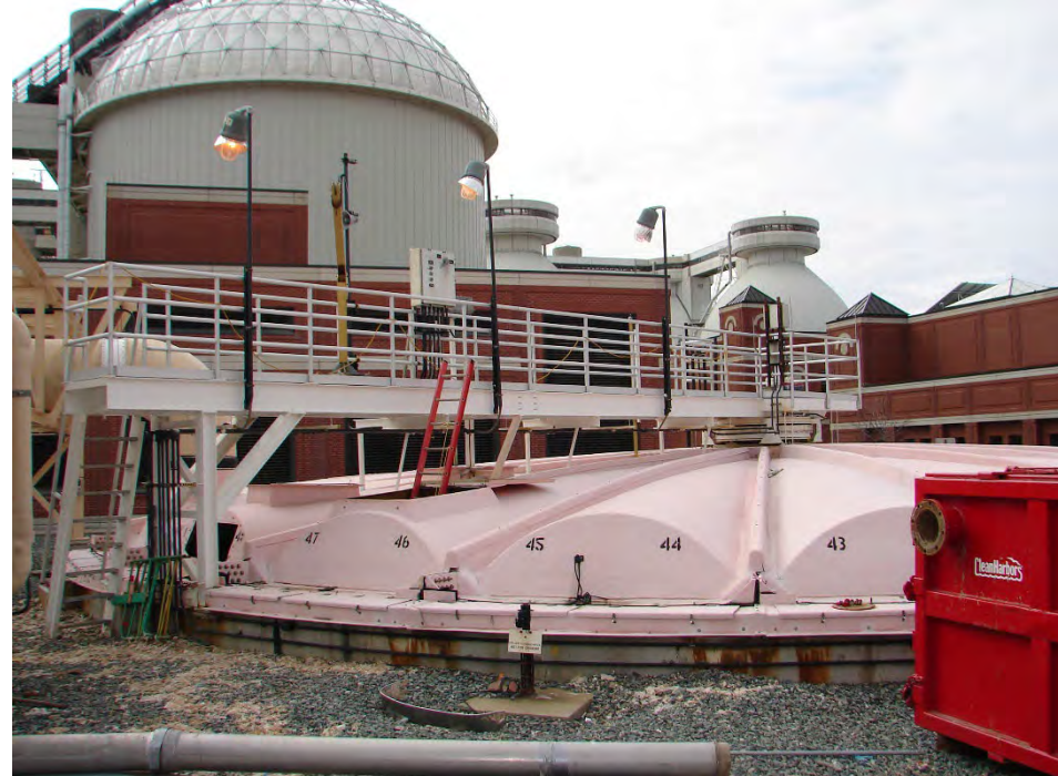
Dig. Gas/Sludge Tank Dome Replacement
