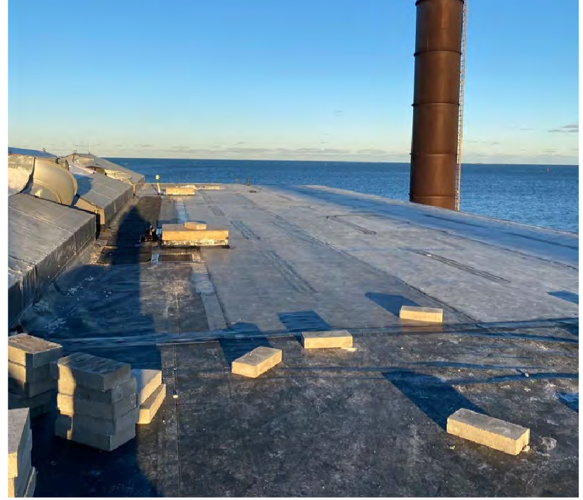
East Odor Control Roof Replacement
