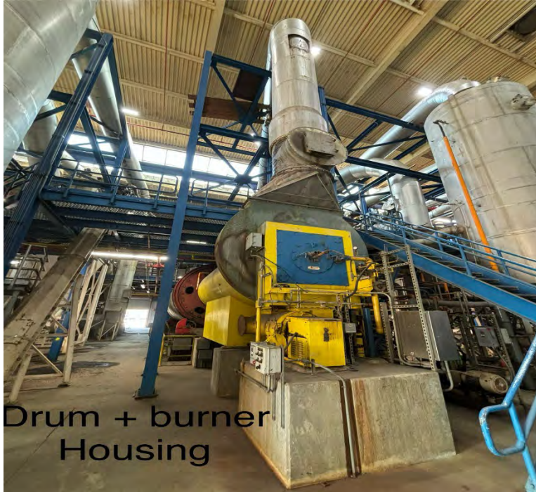
Biosolids Facility Equipment Replacement
