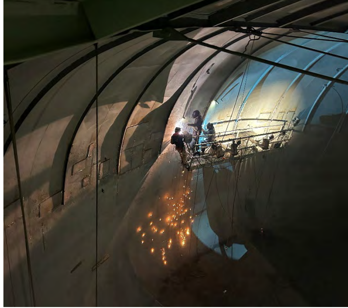
Steel Plate Repairs
