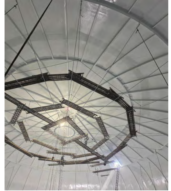
New Internal Tie Rods
