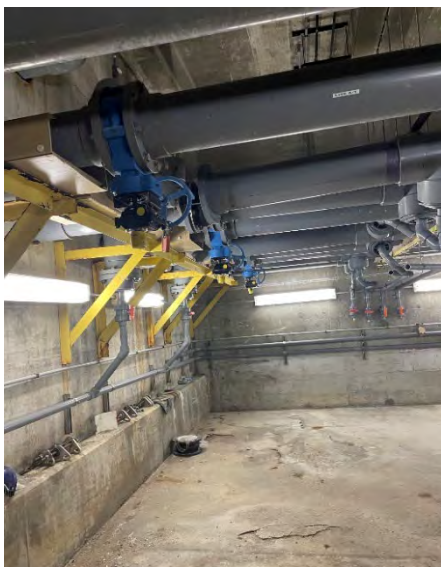
Figure 3- Disinfection Gallery Sodium Hypochlorite Transfer and Return
