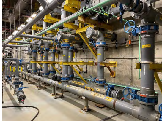
Figure 4 - New 8" Mosite Butterfly Valves Installed by Authority Staff for Reliable System Isolation
