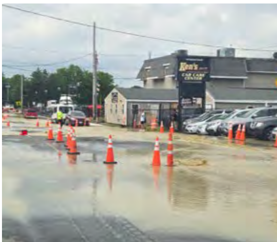
Ballard Street prior to isolation
