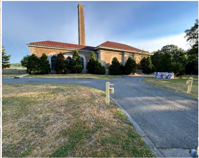
Gillis Pump Station
