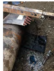
2014 Pine plugs cut and ready for wrap around repair
