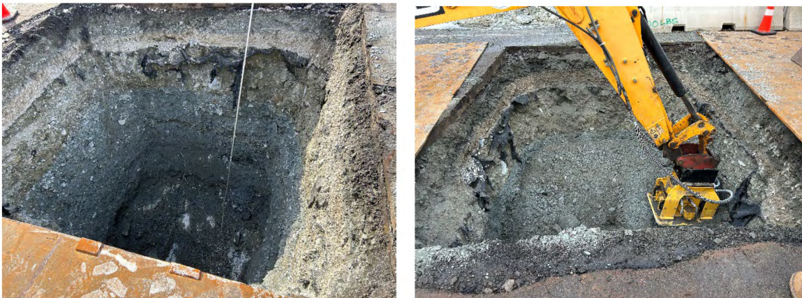
Test Pits in Deer Island Parking Lot 1
