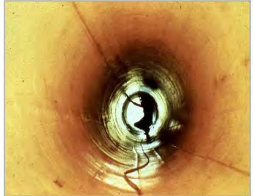
Example of Sewer Rehabilitated with Cured-in-Place Pipe (CIPP) Liner
