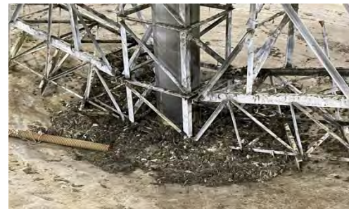
Figure 3. Gravity Thickening Center Column Clog
