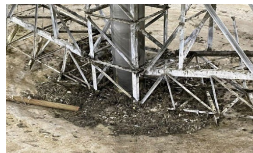
Figure 3. Gravity Thickening Center Column Clog
