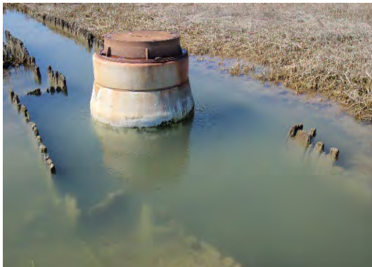
Sewer Manhole in Marsh: Raised and Sealed
