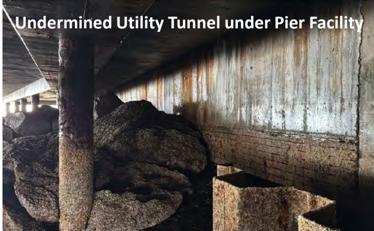
Sinkhole at Pier Facility
