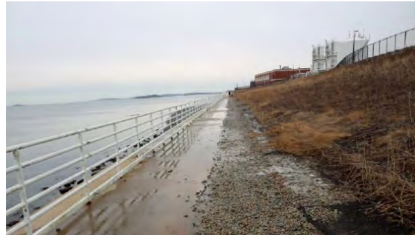
Top of wall/walkway during storm
