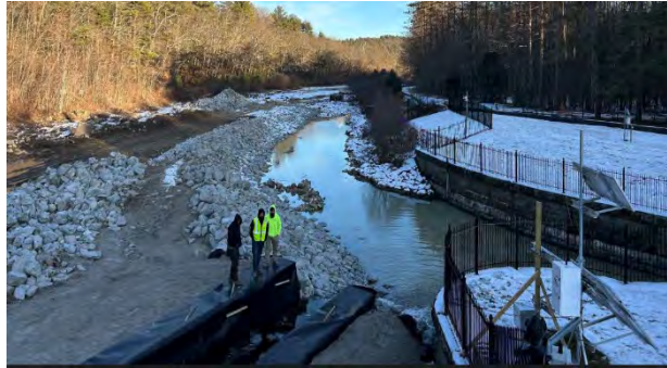
Quinapoxet River Dam Removal
