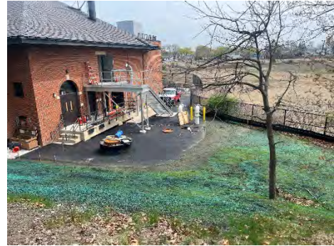
Braintree Weymouth Pump Station
