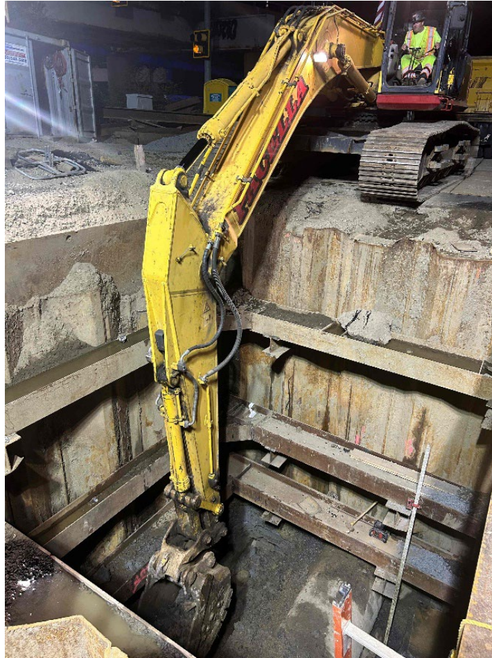
Figure B-1. Excavator at FULL Extension
