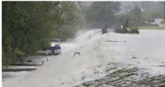
Example of overtopping of earthen dam, Forest Lake, Columbia, S.C., on Oct. 4, 2015
