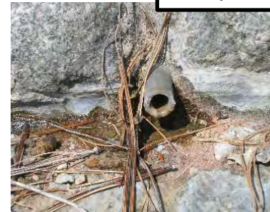
Weep tubes restored
