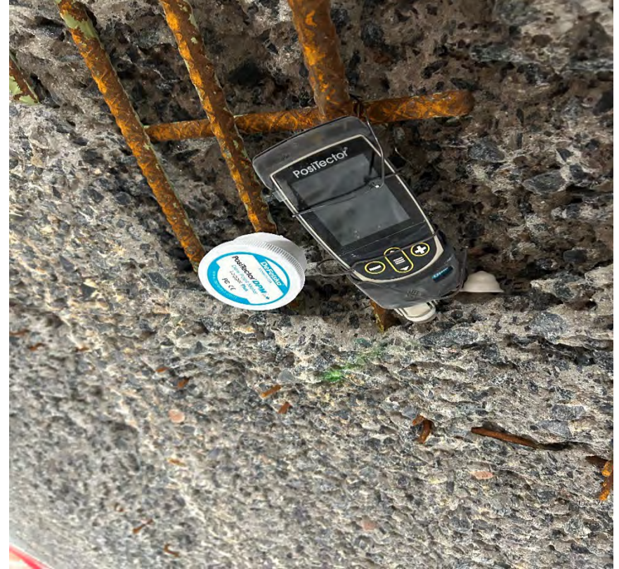
Exposed Rebar
