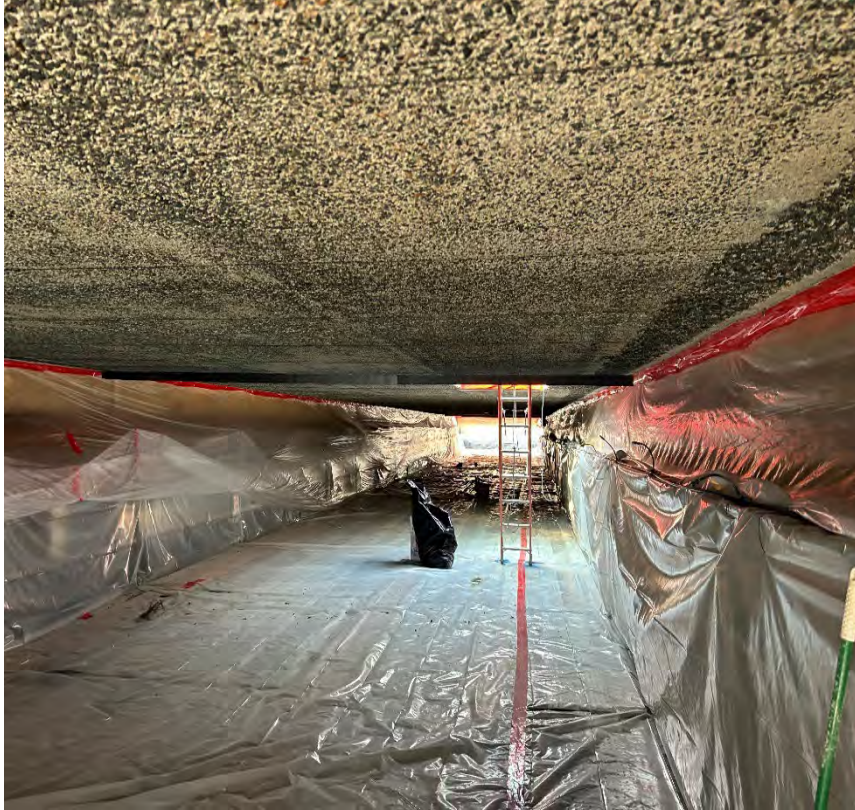
Concrete Cleaning (hydro blast)
