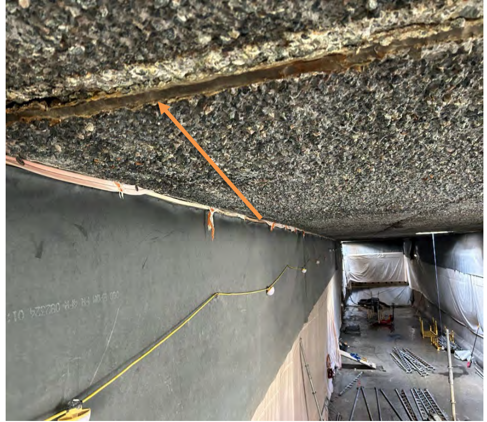
Unexpected Depth of Rebar
