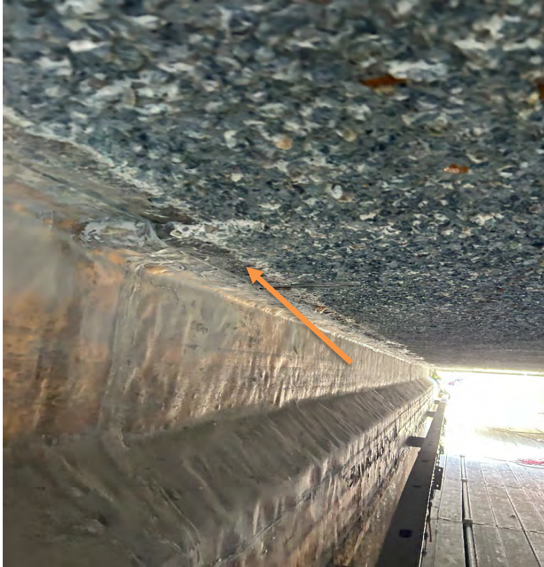
Linabond/Concrete Interface
