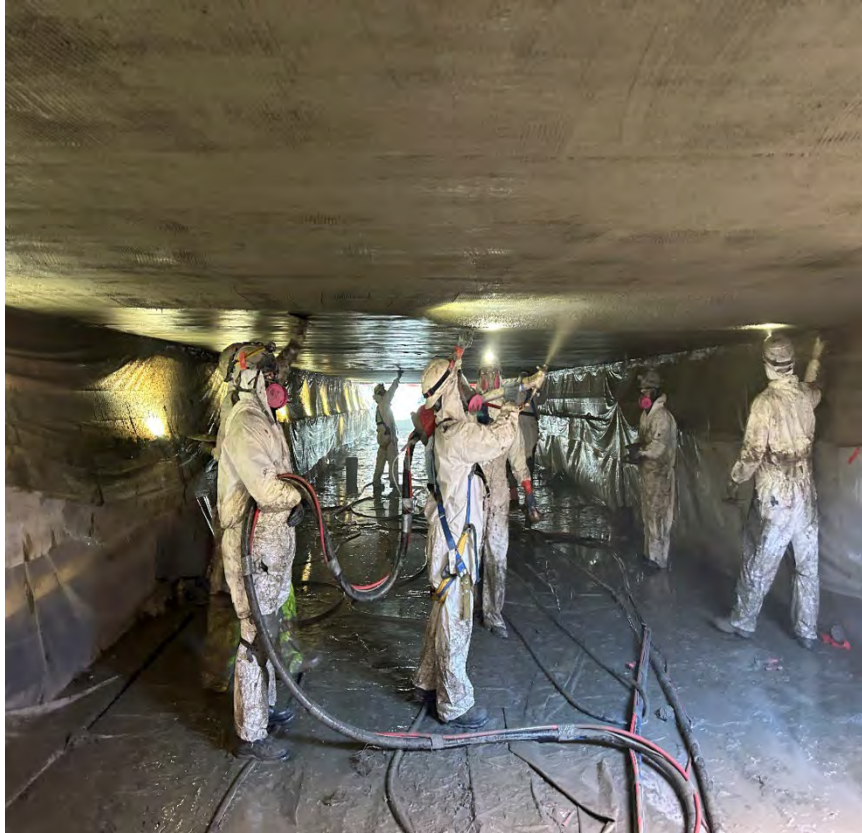
Applying Concrete Resurfacer
