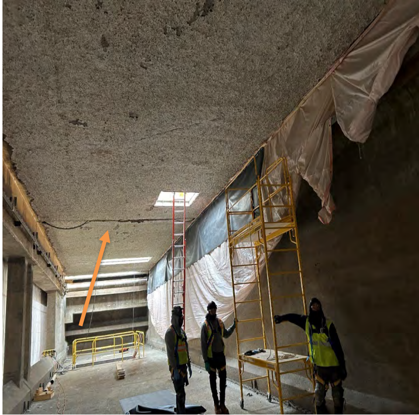
Ceiling Expansion Joint Failures
