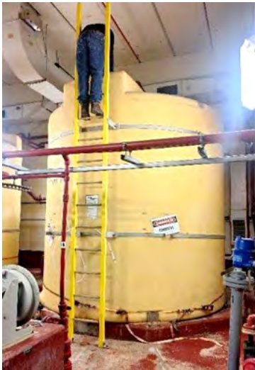
Cottage Farm CSO Facility Sodium Hypochlorite Tank
