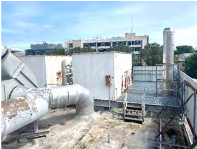
Ward Street Headworks Make-Up Air Handling Units
