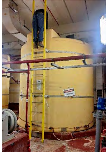
Figure 1: Cottage Farm CSO facility Sodium Hypochlorite Tank
