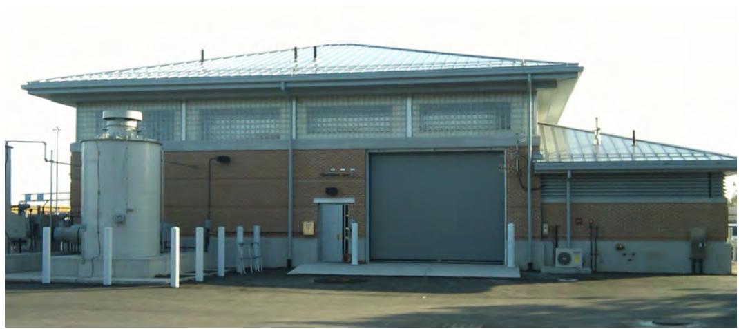
NDB CSO Overflow Pump Station
