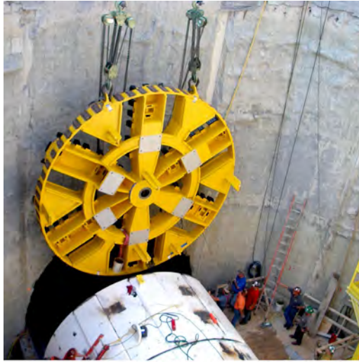
Assembling North Dorchester Bay Tunnel Boring Machine in Mining Shaft, September 2007
