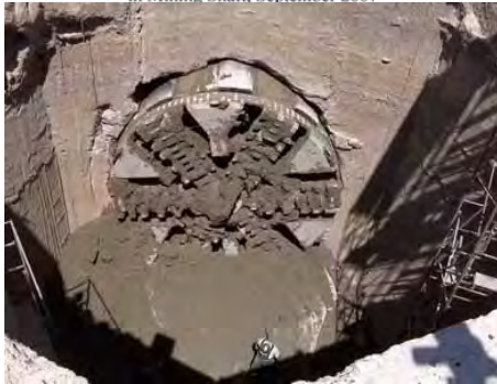
Assembling North Dorchester Bay Tunnel Boring Machine in Mining Shaft, September 2007
