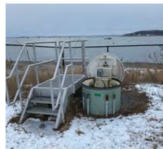
Figure 2: Annual Inspection of a Landfill
