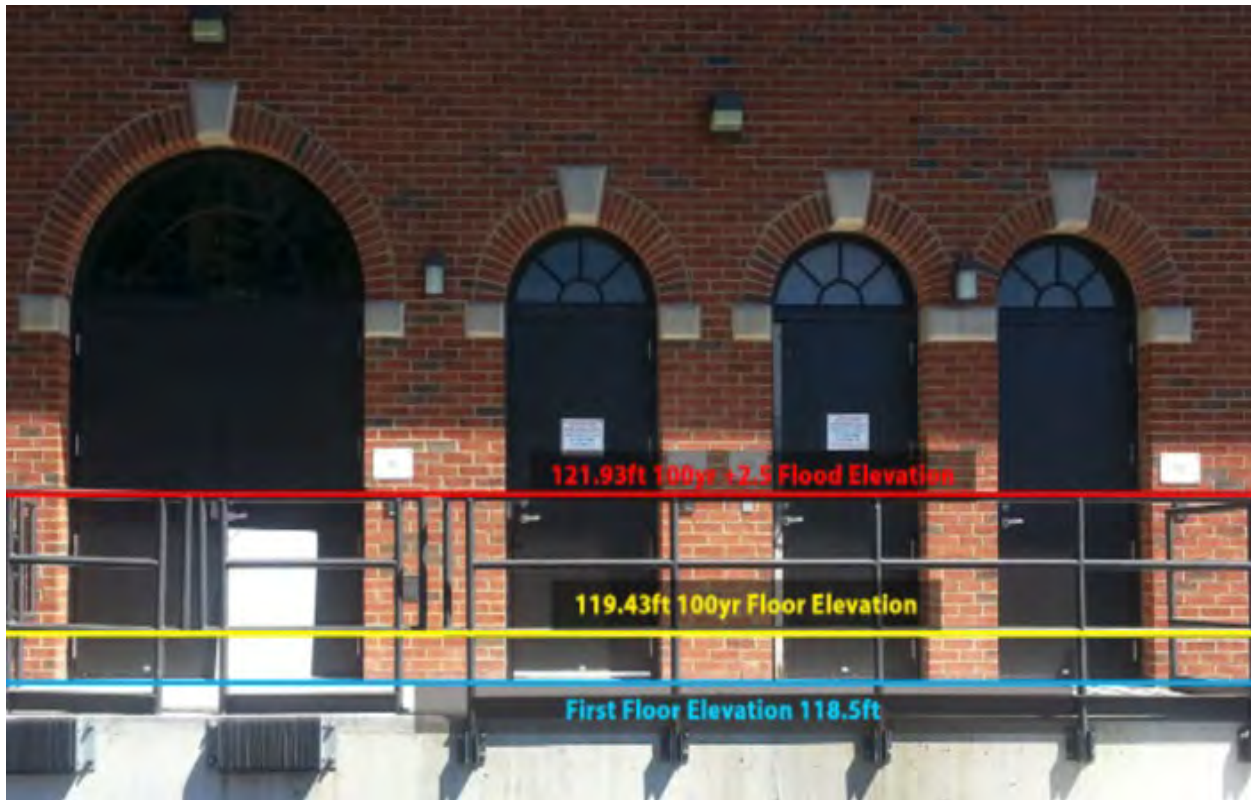
Figure 1: Flood Elevations at Braintree-Weymouth Pump Station
