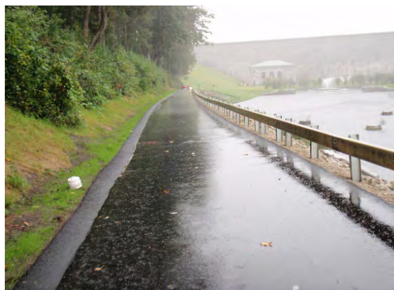
Figure 2. Completed River Road Rehabilitation 2021
