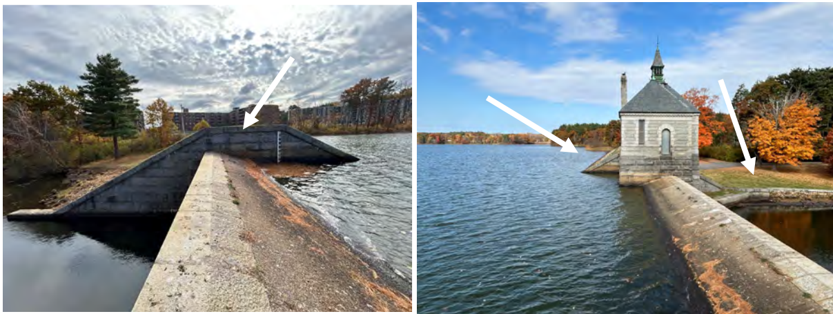
Figure 4. Foss Reservoir Gatehouse and Training Walls Requiring Safety Fencing
