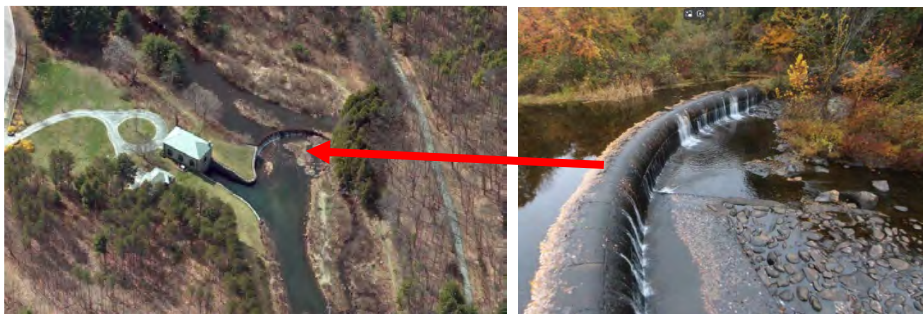
Figure 1. Quinapoxet Dam Before Removal 2024
