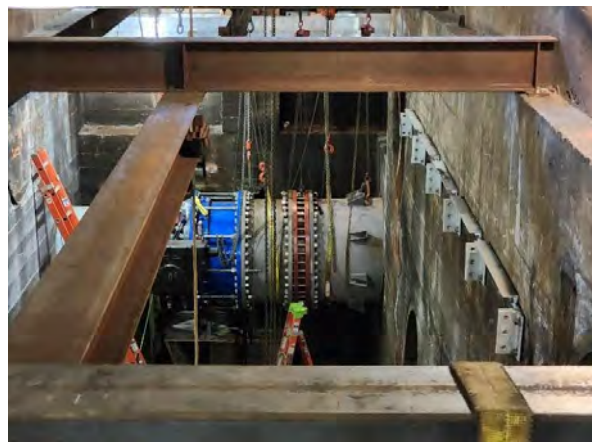
Valve and Piping Installation - Wachusett Dam Lower Gatehouse
