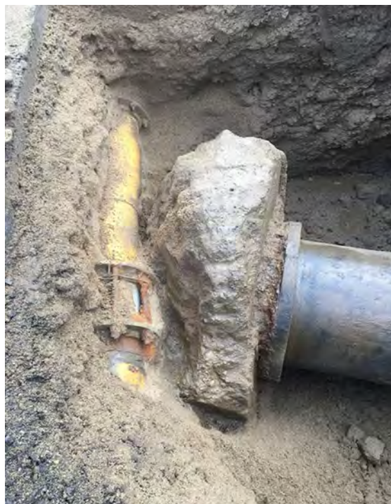
Figure 1: Unapproved removal of thrust block to install gas line, encroaching on MWRA water line and causing a leak
