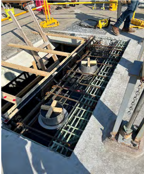
Concrete Slab Extension
