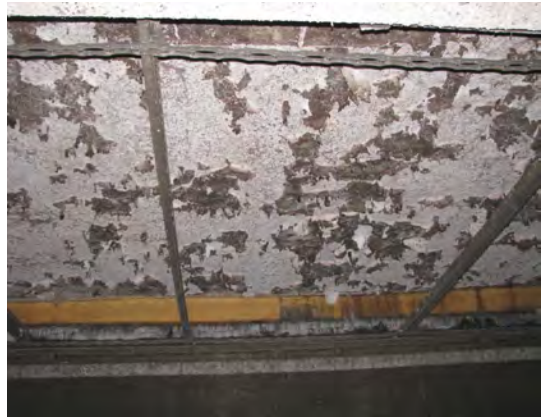
Clarifier Coating Failure
