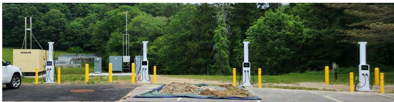
Photo of New Dual Port Level 2 EV Chargers at MWRA Southborough Facility
