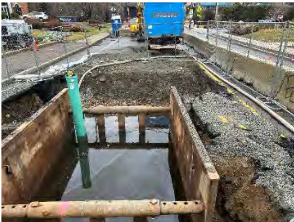
Flooded Excavation from Stream Flow
