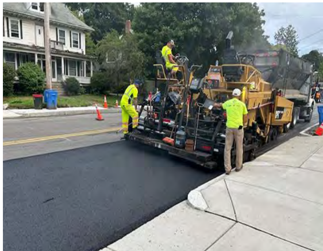
Overlay Pavement on Lexington Street
