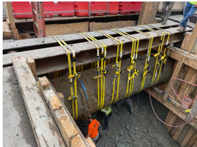
Figure 2: Contractor working with MWRA to properly support MWRA's water main
