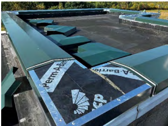
Parapet Installation on Chemical Building
