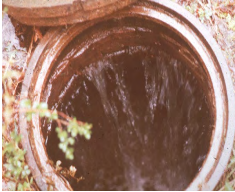
Inflow into a Manhole During Flooding
