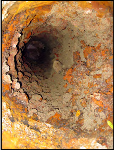
Unlined, Tuberculated Cast Iron Water Main
