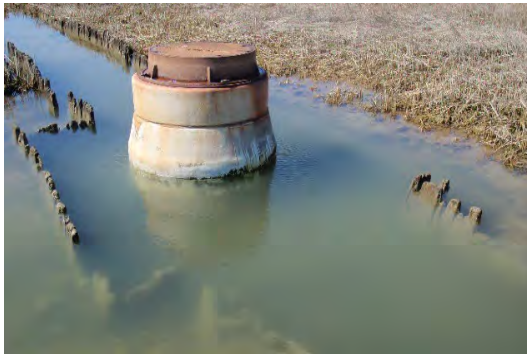
Sewer Manhole in Marsh: Raised and Sealed
