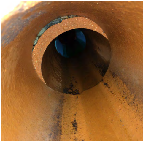
Offset Joint Detected via CCTV Inspection
