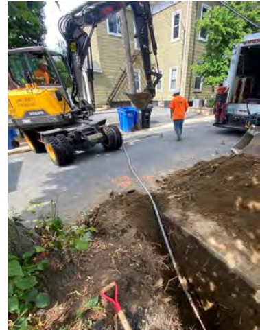
Lead Service Line Replacement
