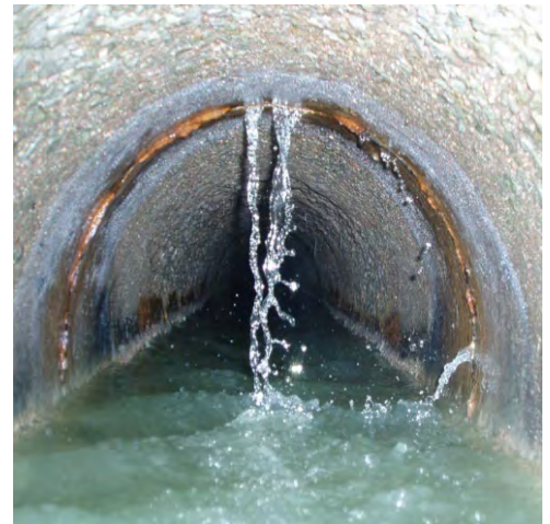
Infiltration into a Sanitary Sewer
