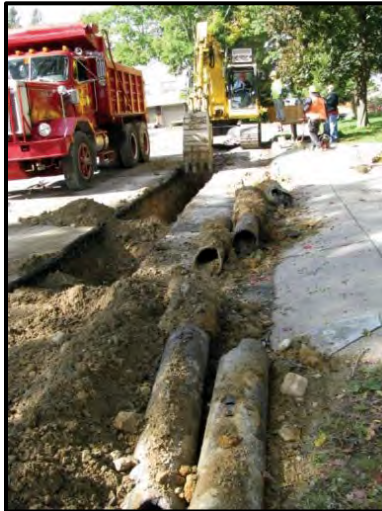
Water Main Replacement Construction
