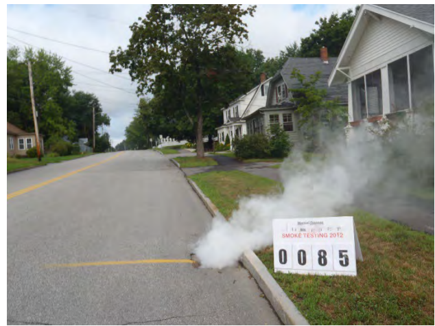
Inflow Source Identified by Smoke Testing
