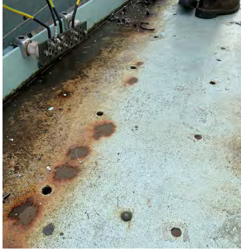
Corroded Exterior Platform
