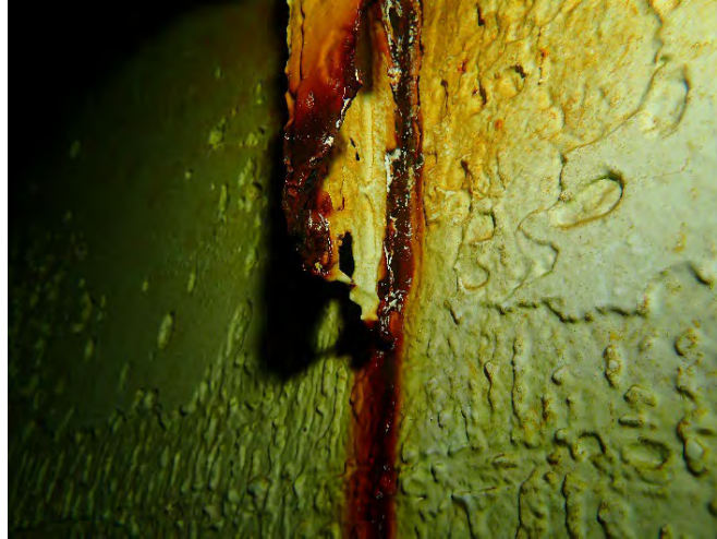
Pitting of Interior Tank Coating
