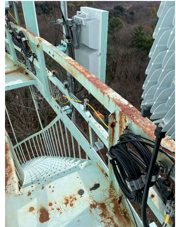
Corroded Guardrail, Stairs & Platform
