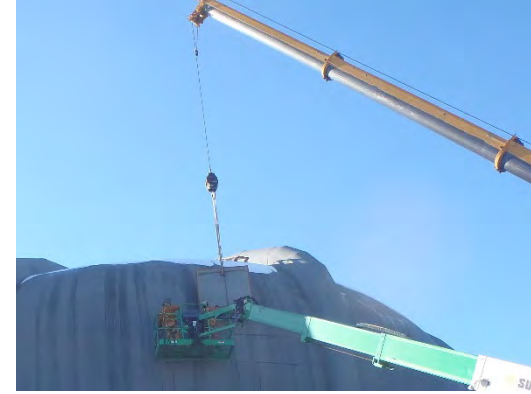
Steel Plate Rigging
