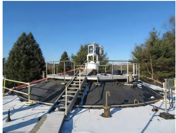
Figure 2 - Digester Fixed Concrete Cover
