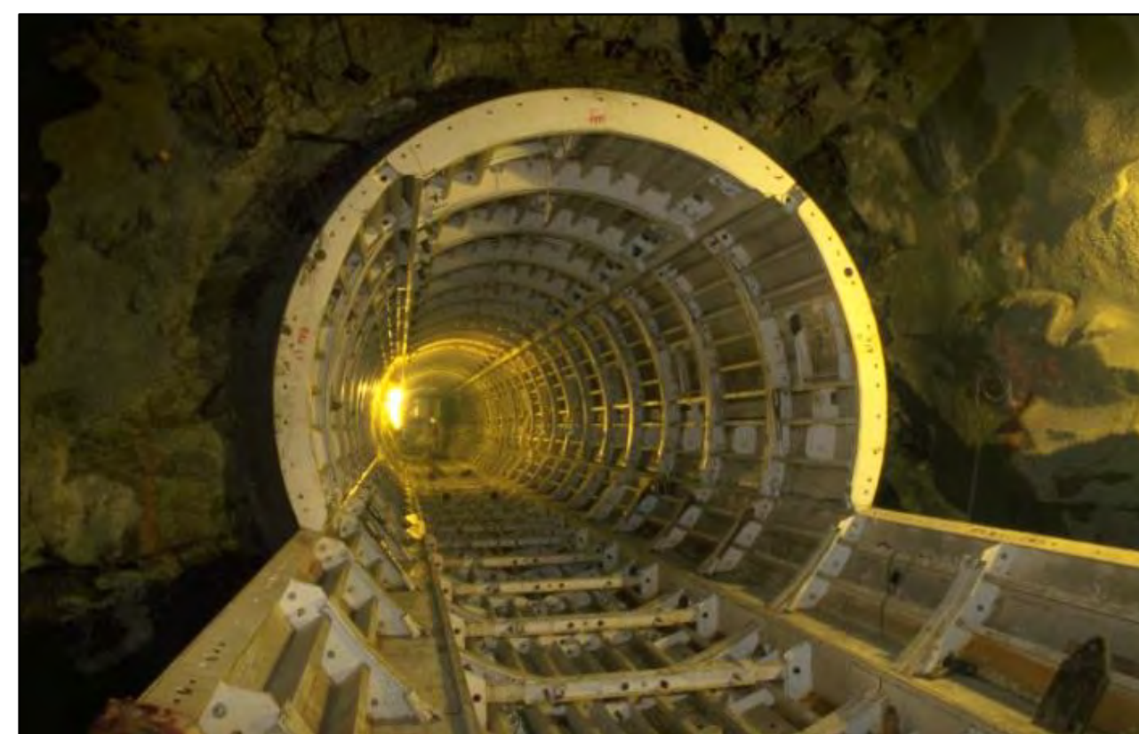
Form for Concrete Lining
