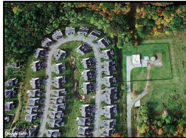
MWWST Shaft L, Framingham
