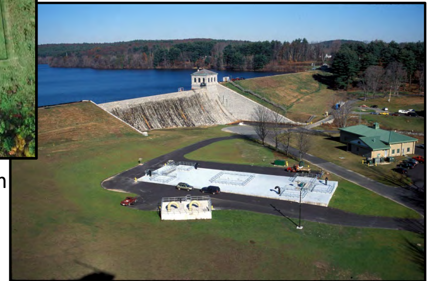
MWWST Shaft E, Southborough
