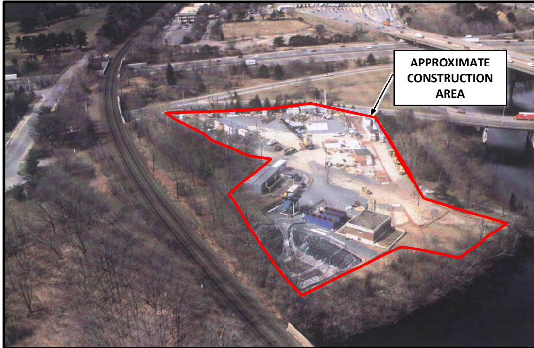
MWWST Shaft 5A – During Construction
