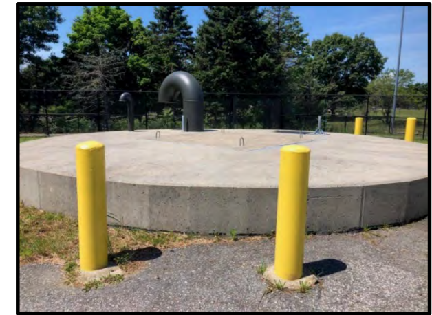
MWWST Shaft 5/5A, Weston
