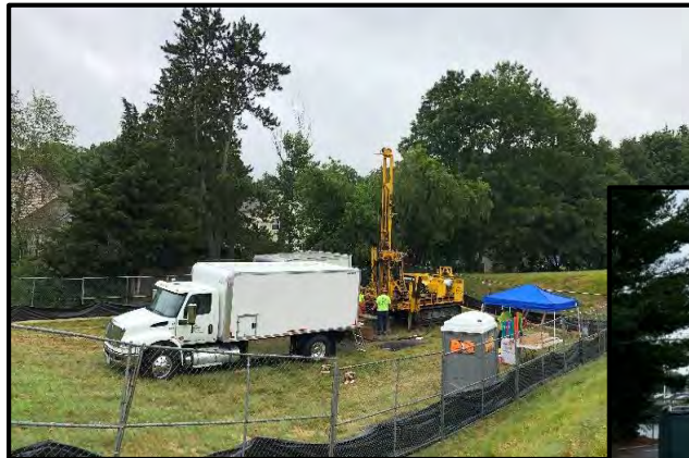
Deep Boring Site Set-up
