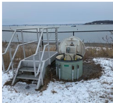
Figure 2: Annual Inspection of a landfill
