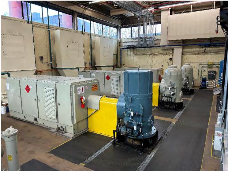
Gas turbine engines with right angle drives
