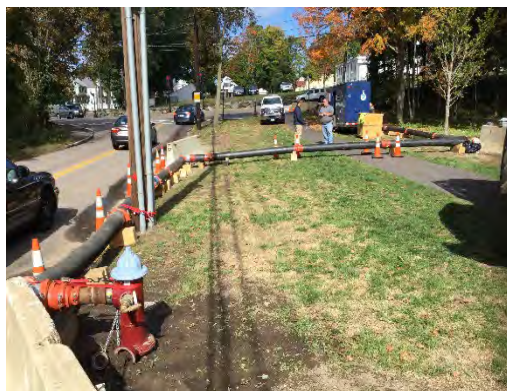
Figure 1: Pumping water from Milton's low service to high service areas
