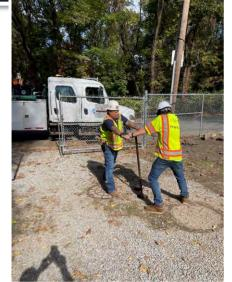
While a repair (using a down hole packer & cement grout) was used to seal the borehole...in record time!
