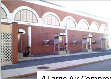
4 Large Air Compressors (2 @ 2,000hp, 2 @ 2500 hp)
