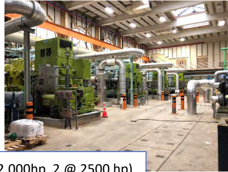
4 Large Air Compressors (2 @ 2,000hp, 2 @ 2500 hp)
