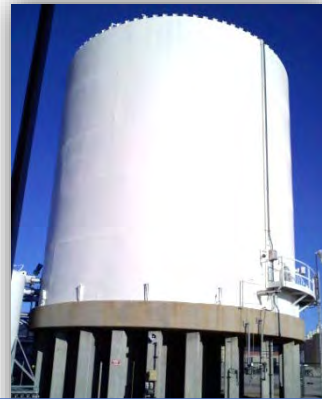
1,000 Ton Liquid Oxygen Storage
