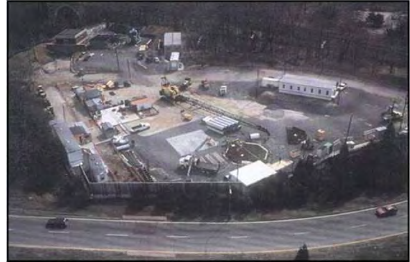
Shaft Site During Construction
