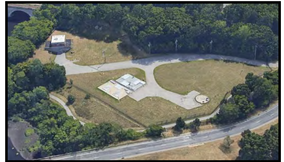
Shaft Site After Construction
