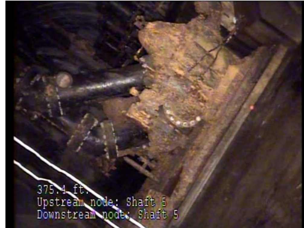
Underground pump room (abandoned with fill)
