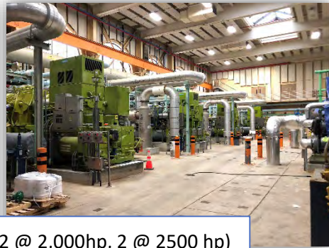
4 Large Air Compressors (2 @ 2,000hp, 2 @ 2500 hp)
