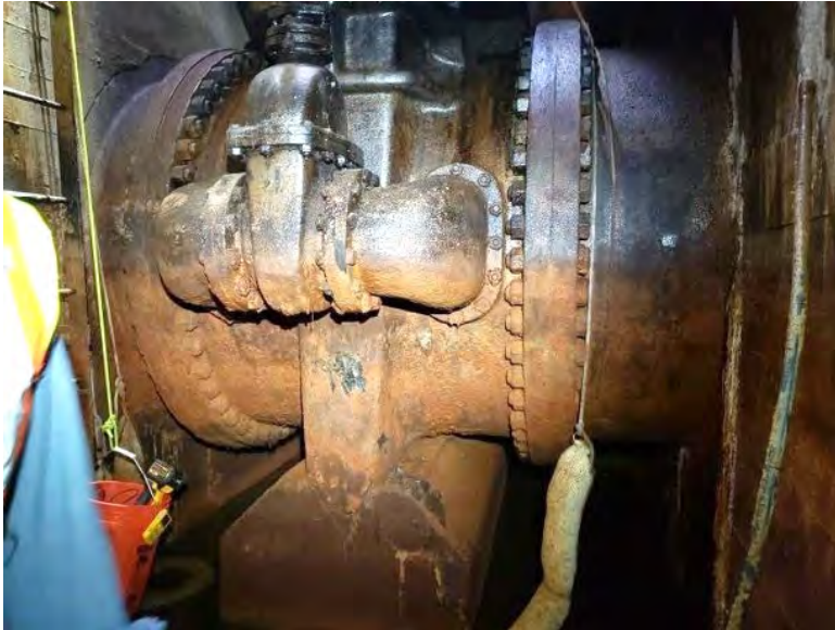
Multiple valve vaults (corrosion protection, bolt replacement, and vault waterproofing)
