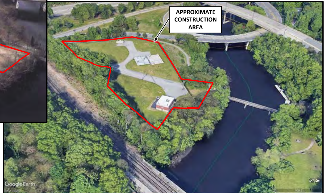
Shaft 5/5A, Weston – Post Construction
