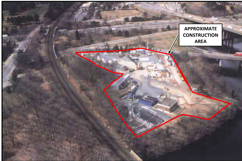
MWWST Shaft 5/5A, Weston – During Construction
