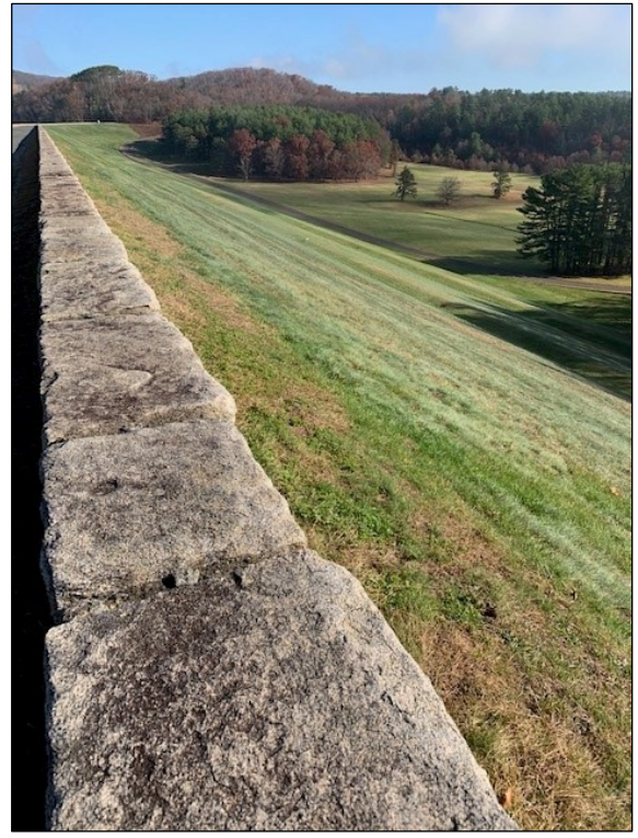
Photograph 4 – Downstream slope of Winsor Dam at Quabbin Reservoir.
