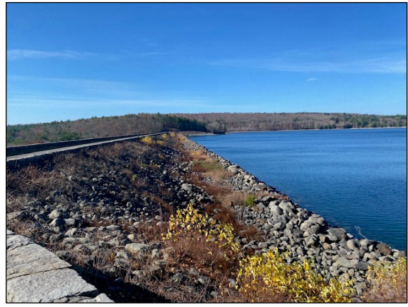
Photograph 8 – Upstream slope of Goodnough Dike at Quabbin Reservoir.
