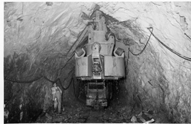
Dorchester Tunnel Raise Bore Shaft
