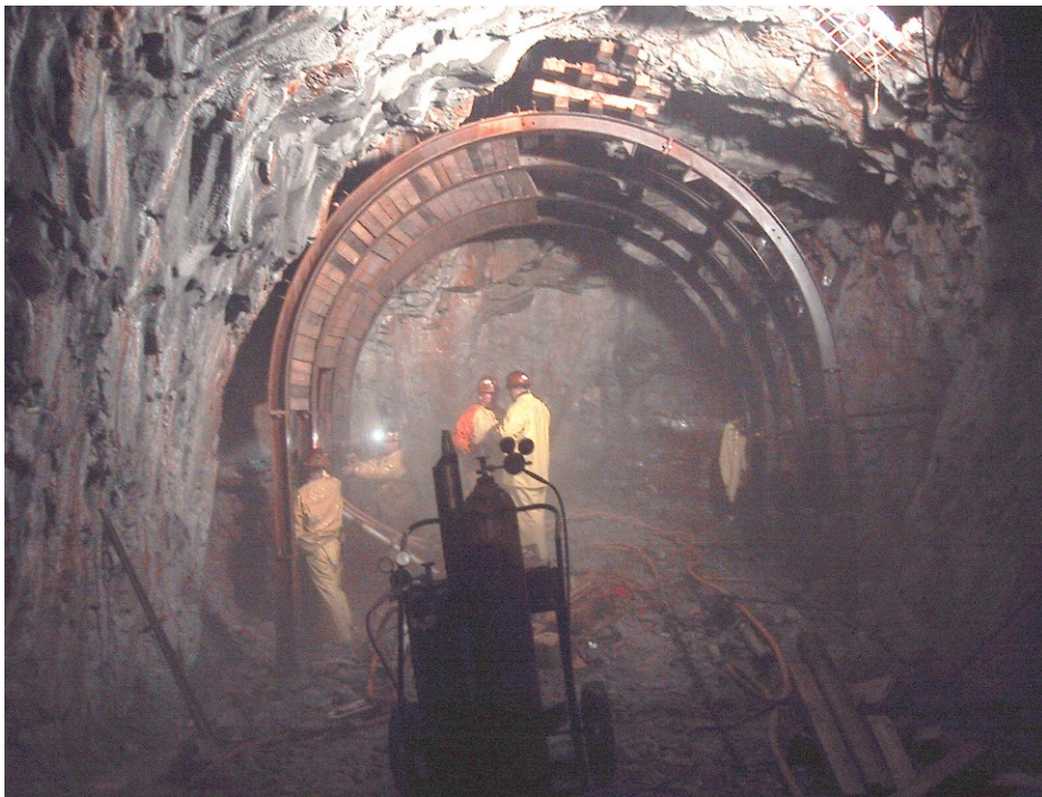
Starter and Tail Tunnels constructed from base of Launching Shaft
