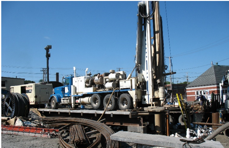
LEFT TOP: Truck-mounted Drill Rig installs pilot hole through top of tunnel.
