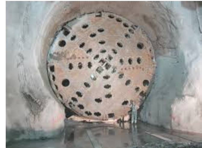
Tunnel Boring Machine (TBM)
