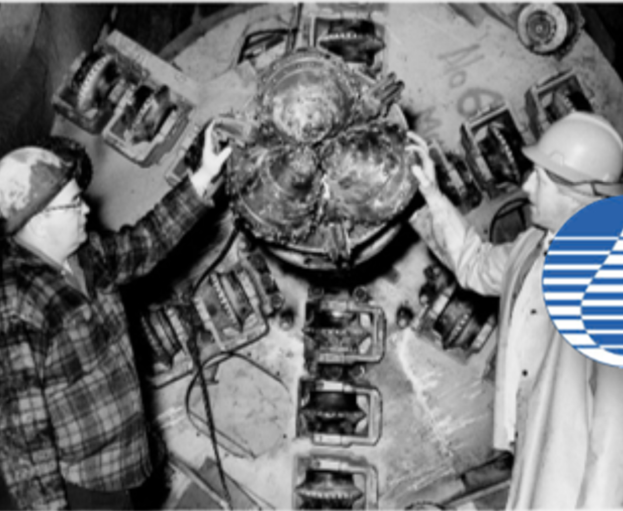
pilot cutters hester Tunnel
