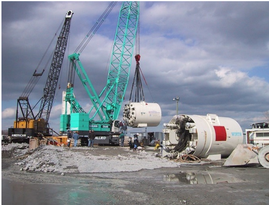
Lower TBM to base of Launching Shaft
