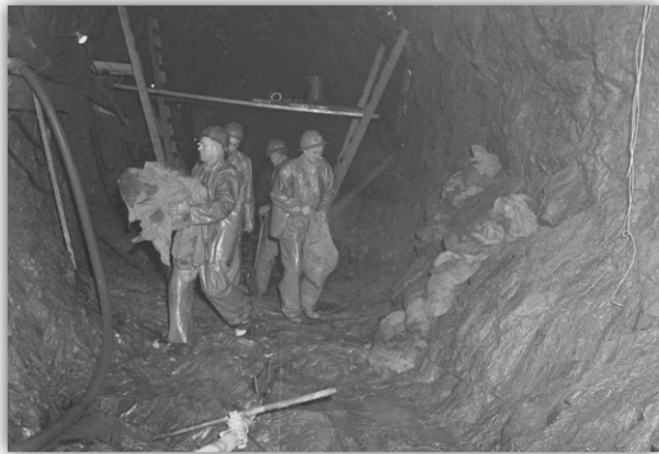
Hand Excavation Drilling & Blasting
